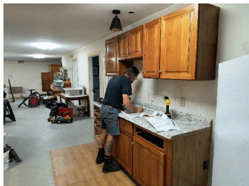
Installing the counter top
